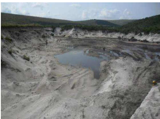
Figure 25. Exposure of the groundwater table by excavation at Mamboukou (Brazzaville).
