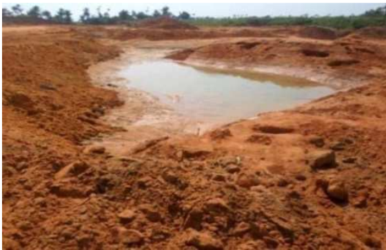
Figure 23. Exposure of the groundwater table by excavation (Côte Matève).
